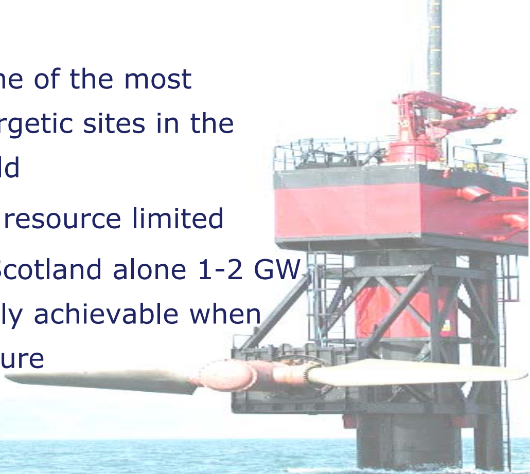
Seaflow (300 kW) by Marine Current Turbines Ltd now in service for 3 years. Twin propeller system deployed later this year
